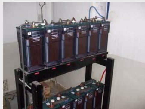
Battery String, Lead-Acid (Vented)
