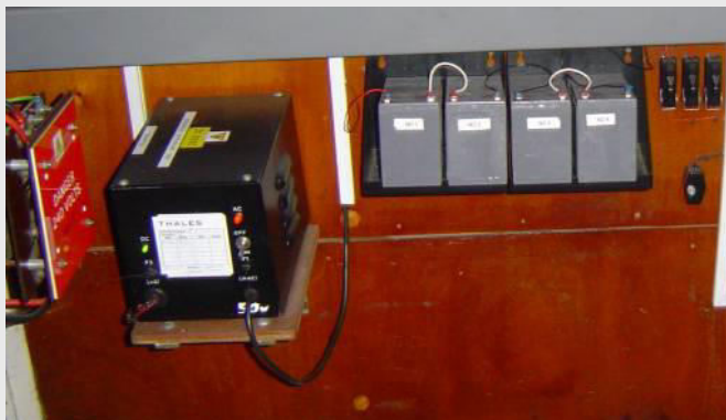
Battery Bank, Lead-Acid (Sealed)
