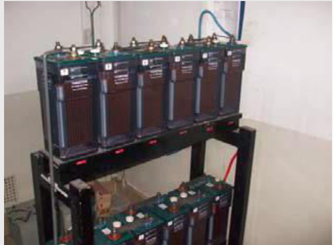
Battery Bank, Lead-Acid (Vented)
