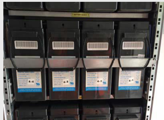
Battery String, Lead-Acid (Sealed)
